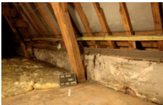
Facade avant, UC040_0211. Photo, S. Modrie © SPRB.
