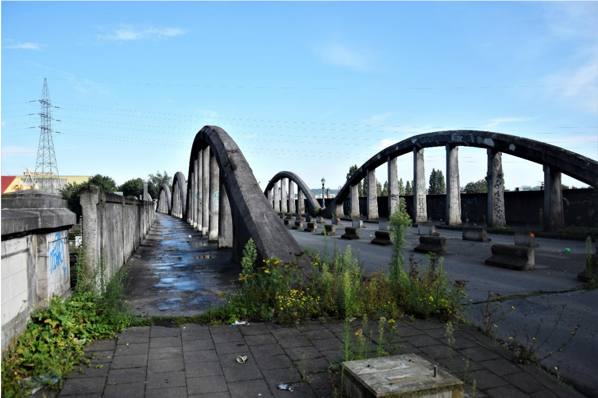
Superstructure, photos CRMS, 07-09-2024
